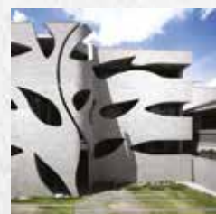
CURVILINEAR FACADE AND BUILDING ELEMENTS
